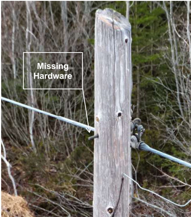
Figure 1 Missing hardware
