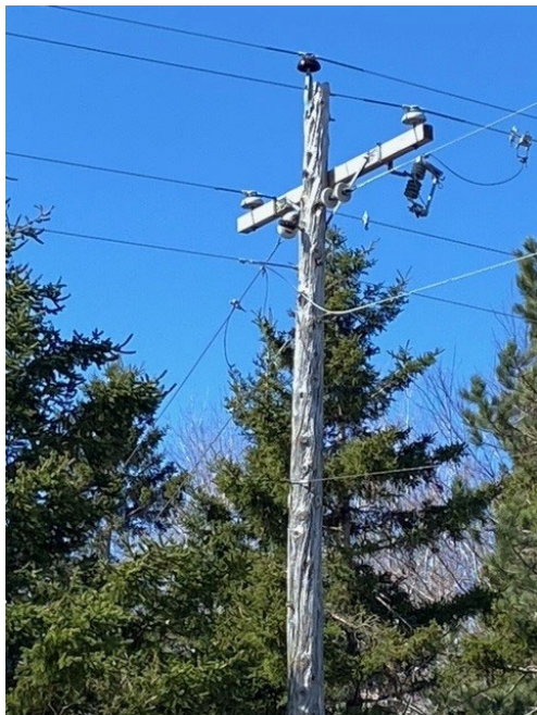
Figure 2 Deteriorated pole
