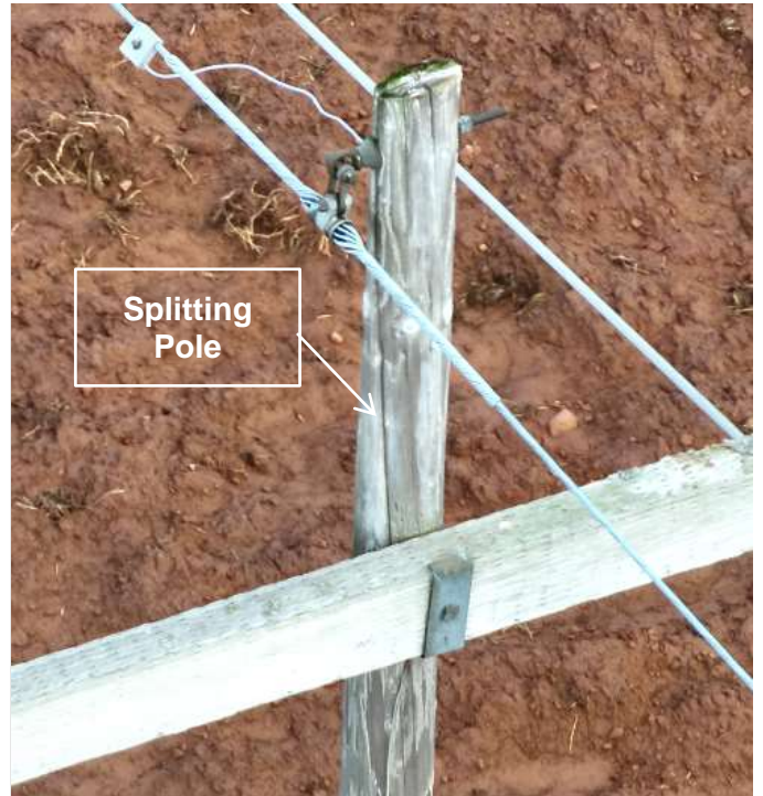
Figure 2 Splitting in the pole
