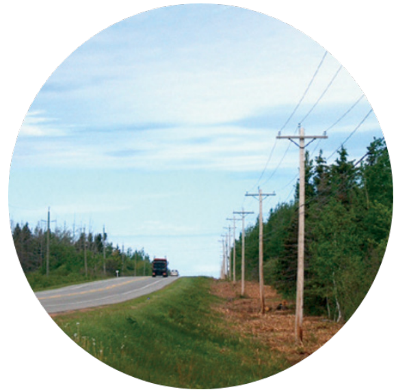
Vegetation and trees have been cleared from power lines to ensure correct distance and safety requirements are in place.
