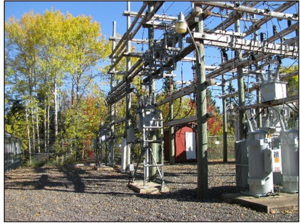
Figure 8: Wood Substation
