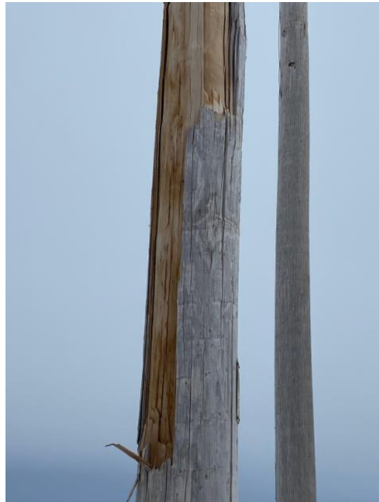
Wood is splitting on pole.
